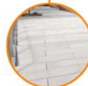
High SRI Hard-scape & Roadway Paving
